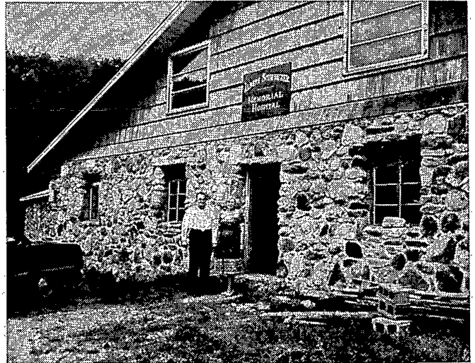
A hospital being built on faith, hope and human concern
